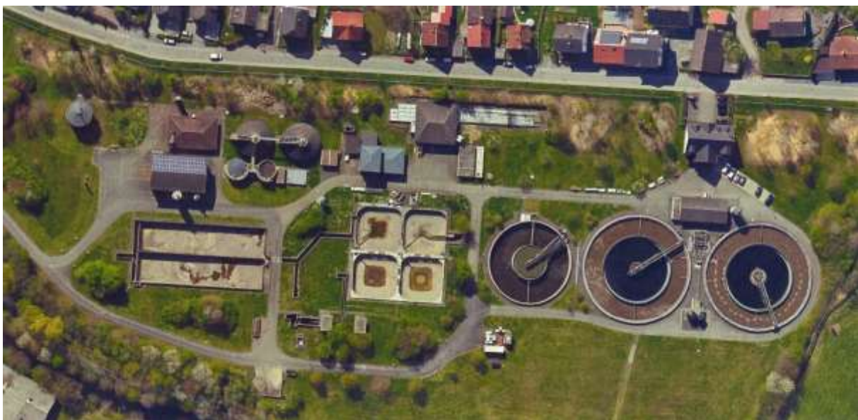
Picture 1 WWTP Asselbrunn, Abwasserverband Mittlere Mümling
